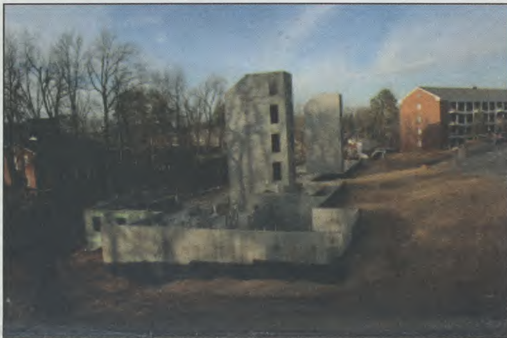
CONSTRUCTION PROGRESSES ON BLESSING HALL
